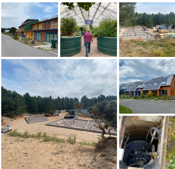
Views of the new development during construction
